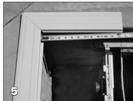
5 Measure and cut the lid panels (X0048), C-cap (X0053), and hinge attachment (X0940) approximately 1 1/4 in shorter than the actual width to the inside of the lid end supports. This allows space for the cut cover and lid wedges to attach to the ends of the lid panels to cover any cuts.
