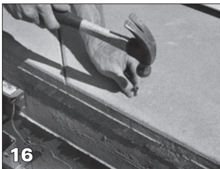
16 Remove the lid and hammer the plastic anchors (A1706) into the holes.
