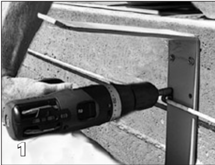
1 Attach the 97 degree angled brackets (A2430) to the back wall of the housing 1 in below the top of deck.
