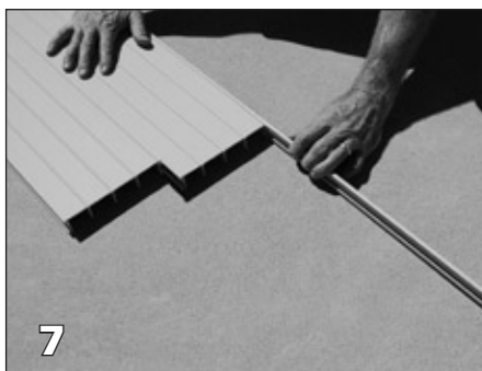
7 Slide the lid panels (X0048) and C-cap (X0053) together.
