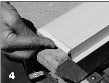
4 Insert the end caps (A2426) to the lid end supports.
