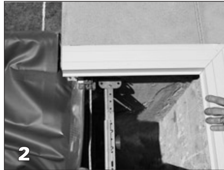
2 Set the lid end support (A2429) in the ends of the housing in order to get an accurate measurement for the lid panels.
